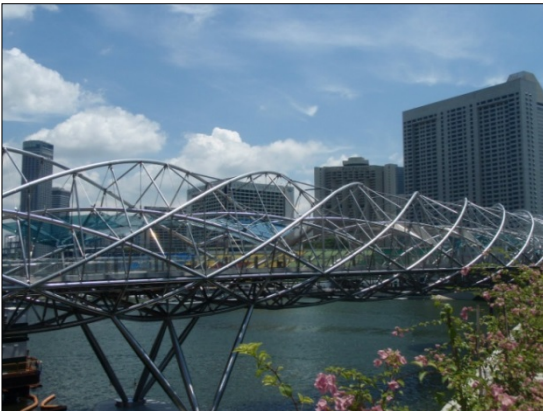
Helix Bridge, Singapore, 2011
